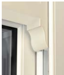
Run-through Sash Horn
